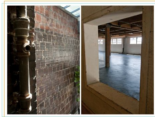
Architectural details and oddities were left in place, rather than hidden.
