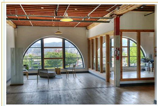
Original rounded windows were not only left intact, they were improved on, giving occupants full daylight indoors.
