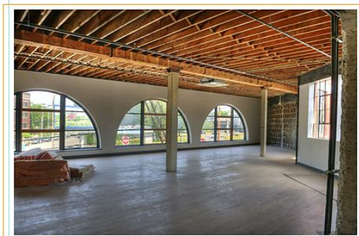
Original joists strengthened by newer beams.
